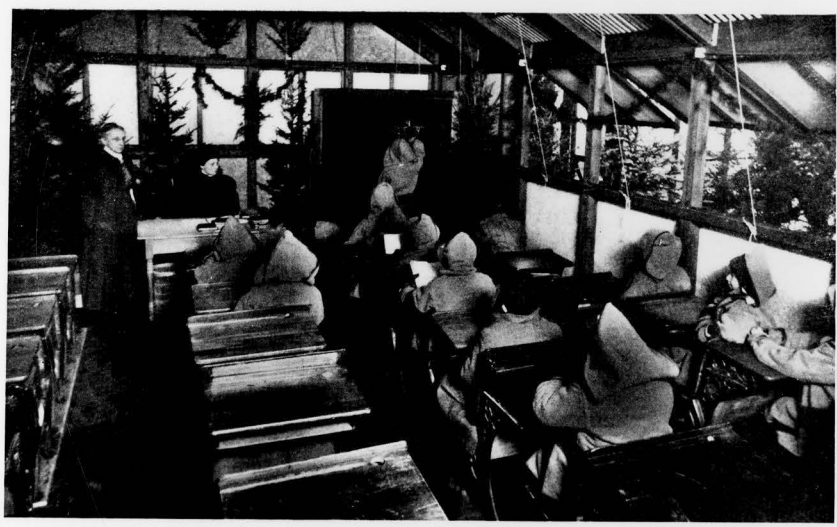
Photograph of the Chicago roof tent, as published by The Survey , to illustrate permanent construction
