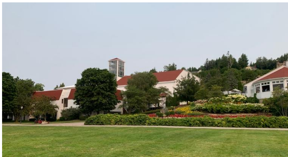
Figure 18. Since the 1950s, the unassuming Mission House has been dwarfed by the Mission Point Resort complex, which was originally built by Moral Re-Armament and later used as an evangelical college. Photo by the author.
