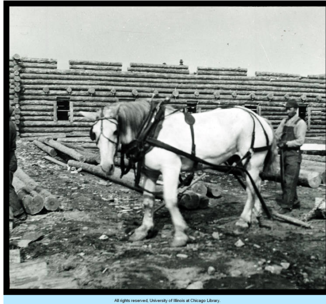
Figure 10. A man works with a draft horse to construct the Old Fort Dearborn replica. COP_17_0025_00000_033, Century of Progress Records, Special Collections and University Archives, University of Illinois at Chicago Library.
